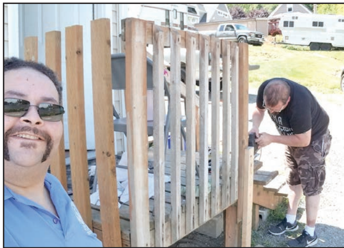
Above: Adrian Camez, Levi Wilson and Mike Hill (not pictured) repaired a porch for a resident in Everett on July 10.
